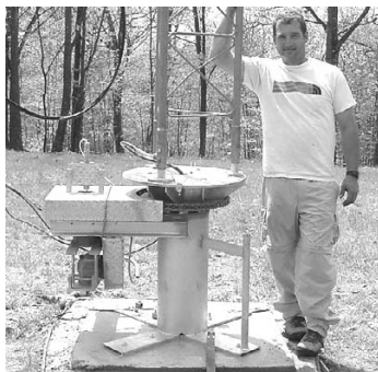
Ground mounted base for 300 feet of Rohn 55G/AB105.
