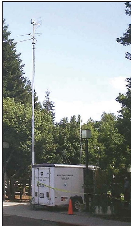
Fig 9.62—FM voice repeater, amateur television (ATV), and HSMM antennas mounted on a hydraulically operated mast. This portable installation was used to provide shared high-speed Internet access and other special communications support to the many hams attending the 2003 Pacificon Hamvention in San Ramon, CA. The HSMM station is also used to provide streaming video or amateur digital video (ADV) to the Mount Diablo ARC's analog FM ATV repeater on the nearby mountain. (Photo: John Champa, K8OCL)
